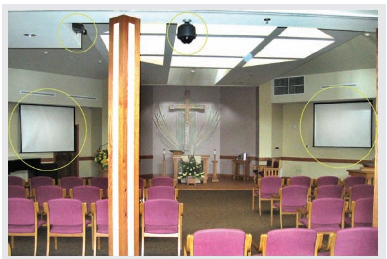
Dual drop-down screens with companion video projectors and video camera to aid in broadcast to shut-ins.
